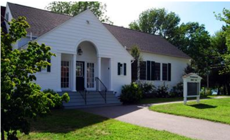
2 North Street, Kennebunkport *
